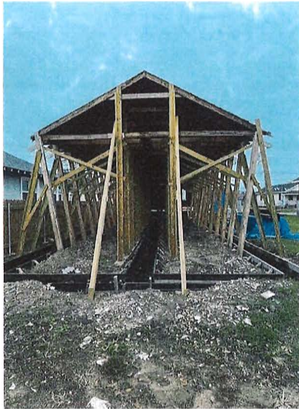
Photograph #3 Lateral Stability Unsafe for Construction Personnel
