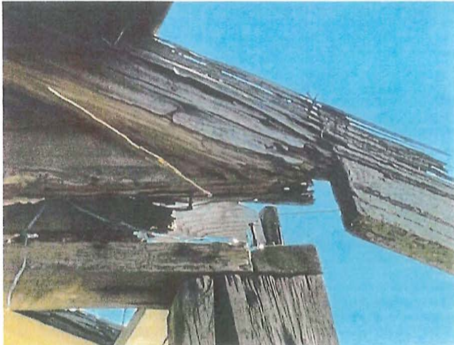
Photograph #8 Roof deterioration is past repair and in need of replacement.
