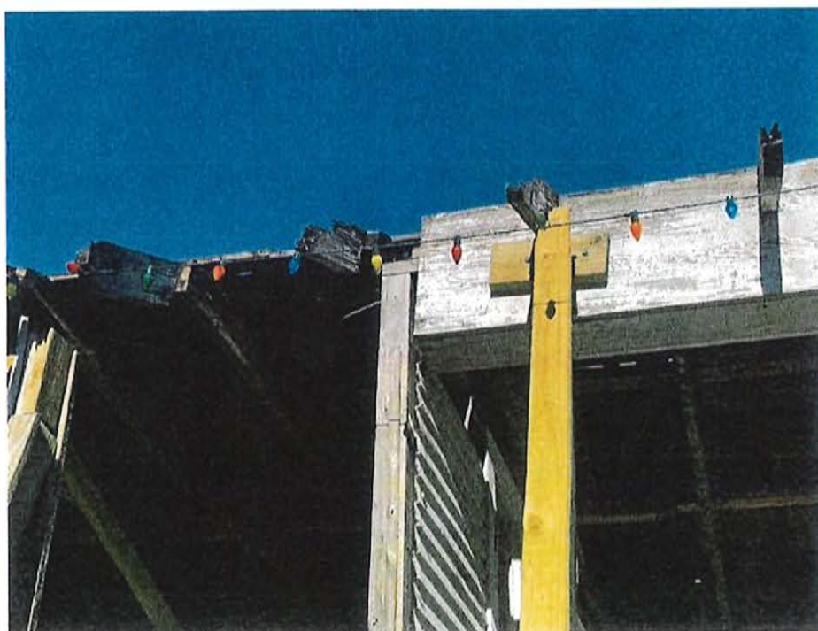
Photograph #4 Collar Braces and Rafters in Poor Condition
