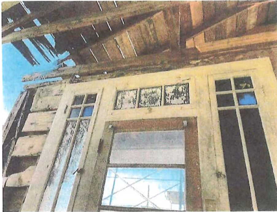
Photograph #1 Portion of Front Façade i.e., Millwork and door frame can be salvaged. Supporting framework is in disrepair and in need of replacement
