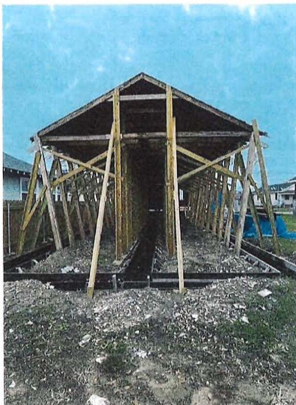
Photograph #3 Lateral Stability Unsafe for Construction Personnel
