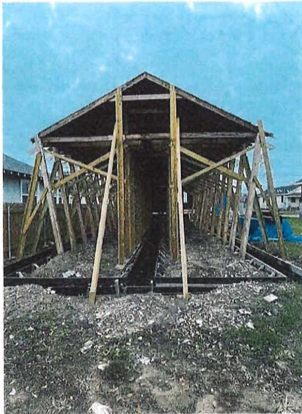
Photograph #3 Lateral Stability Unsafe for Construction Personnel
