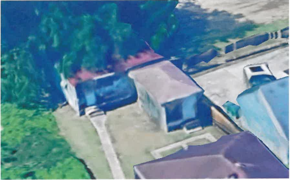
Photo 3 – Bird’s Eye View of Large & Small Sheds. Small shed will remain.
