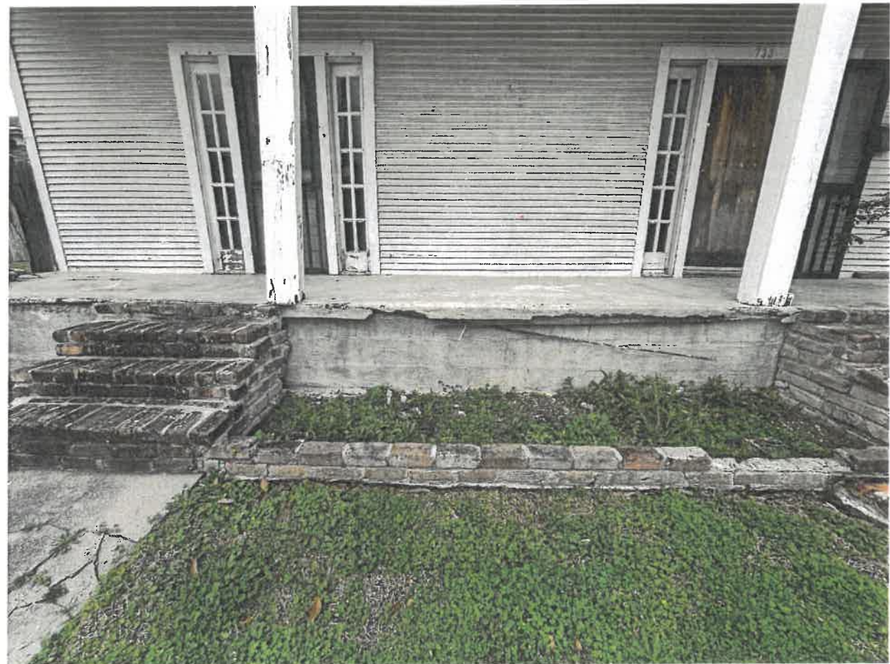
6 th Street Elevation – failing porch slab and compromised columns
